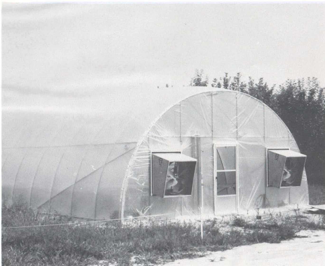
The small greenhouse shown above was constructed by the Cheasapeake Corporation of Virginia in order to grow containerized genetic test seedlings.
