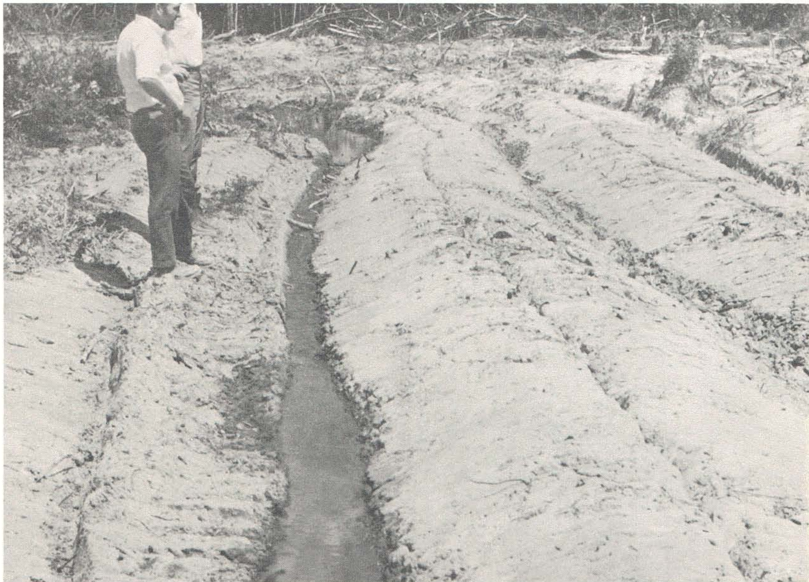
Intensive site preparation is becoming more common, even on drier sites. Shown are beds on a sloping Piedmont ridge in Alabama on lands of Hammermill Paper Company. Such beds, made on the contour, result in catchment of water that would normally be lost.
